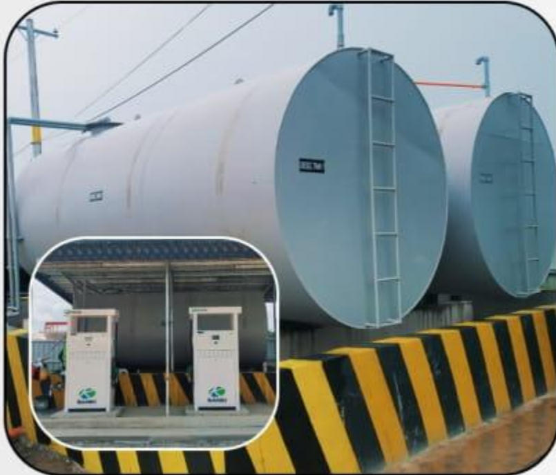
ACCIONA DAELIM FUEL STATION
